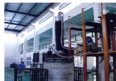
252kV/3150A套管在温升实验 Bushing 252kV/3150A in heat run test
